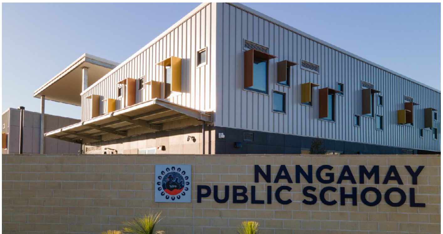
Image: Nangamay Public School, which recently achieved a 4 Star Green Star Buildings certification.
